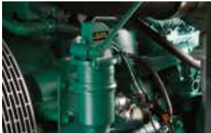
Lube oil drain pump
